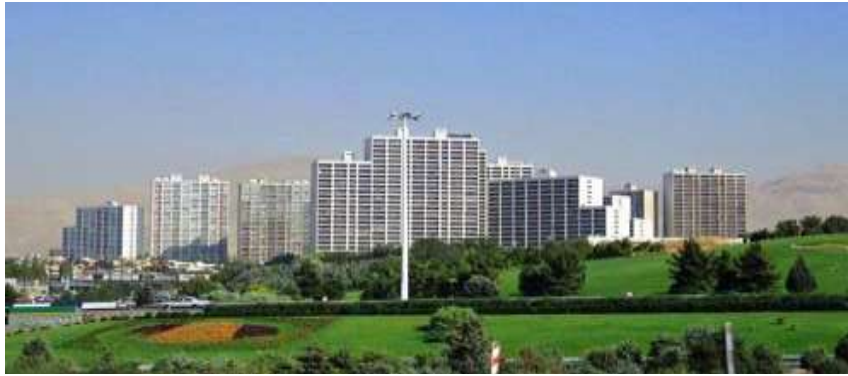
General view – Sanat Square, Ekbatan town, Tehran
