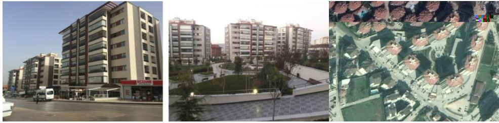
Figure 12. Photographs taken from the Sample E Figure 13. Aerial photo of the Sample E
