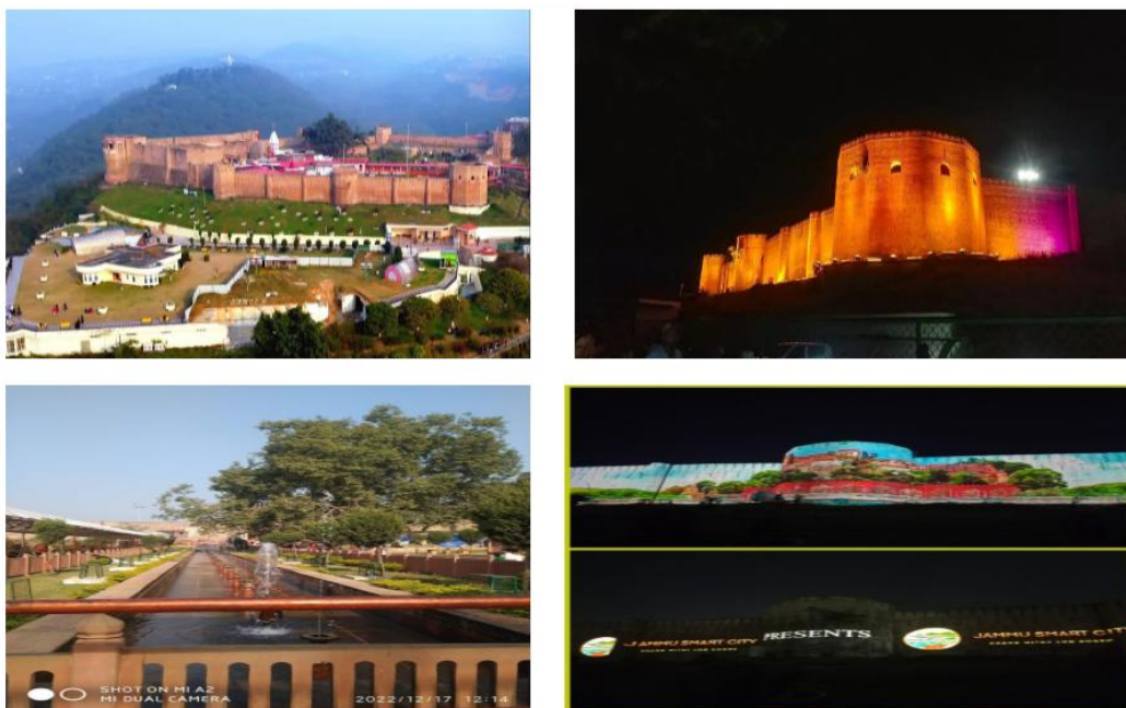
4. Images from left to right show us the aerial view of the ancient Bahu fort –Jammu, its restoration and Adaptive Reuse i.e. Beautification of Landscape, Illumination and Light and Sound Project, Jammu, Image Source: Monika Choudhary
