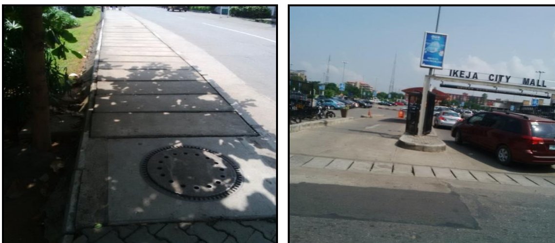
Figure 7: Showing closed and well planned drainage system toward Alausa secretariat (Source: Personal archive of author, 2014).
