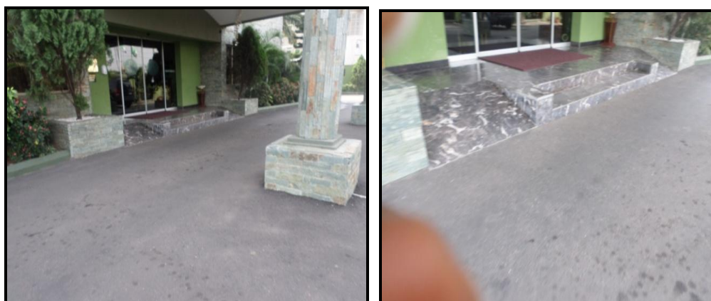
Figure 15: Showing inadequate ramp slope and slippery floor finish at renaissance hotel along the sampling area (Source: Personal archive of author, 2014).
