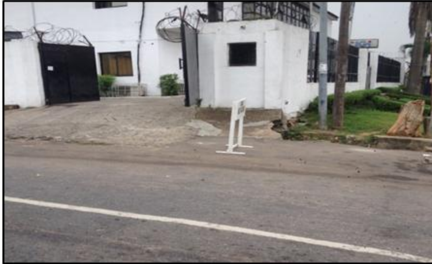
Figure 16: Showing entrance to the IGI building with a steeply deformed ramp access (Source: Personal archive of author, 2014).
