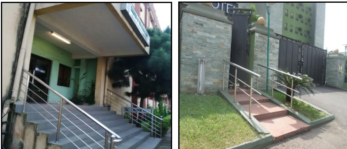
Figure 6: Showing guard rail of 1200mm height on steps of renaissance hotel and state secretariat building (Source: Personal archive of author, 2014).
