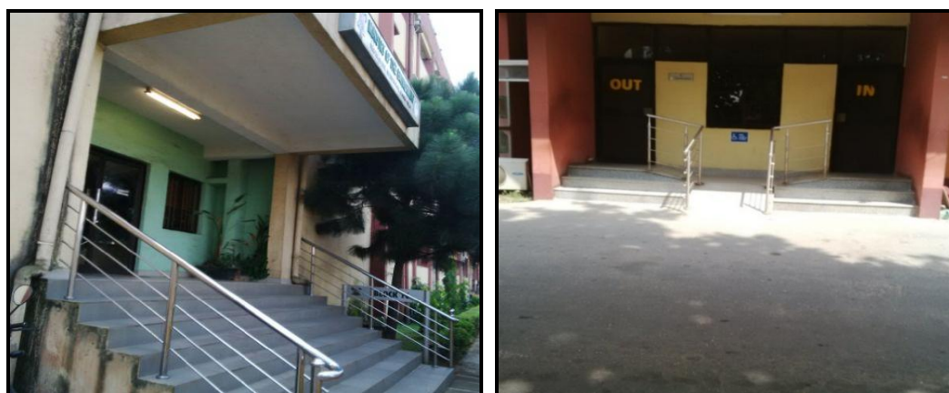
Figure 14: Showing Lagos State Secretariat inaccessible entrance to disabled people along the sampling area (Source: Personal archive of author, 2014).
