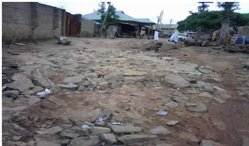
Plate VI: An erosion-threatened access road filled with stones and solid tar materials at an Informal neighbourhood along Top Medical Rd
