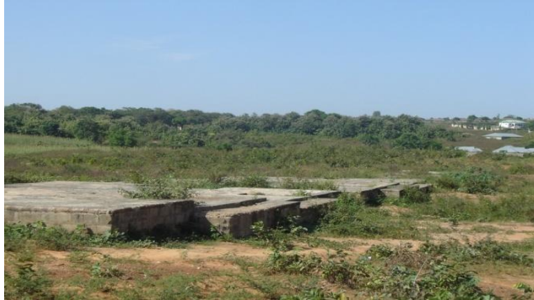
Plate II: Abandoned Penil Estate by CE-DEV Global Ltd Source: Google Earth, 2009.
