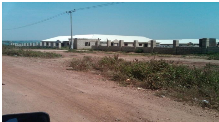
Plate III: Ongoing construction opposite NECO Head Office, Minna
