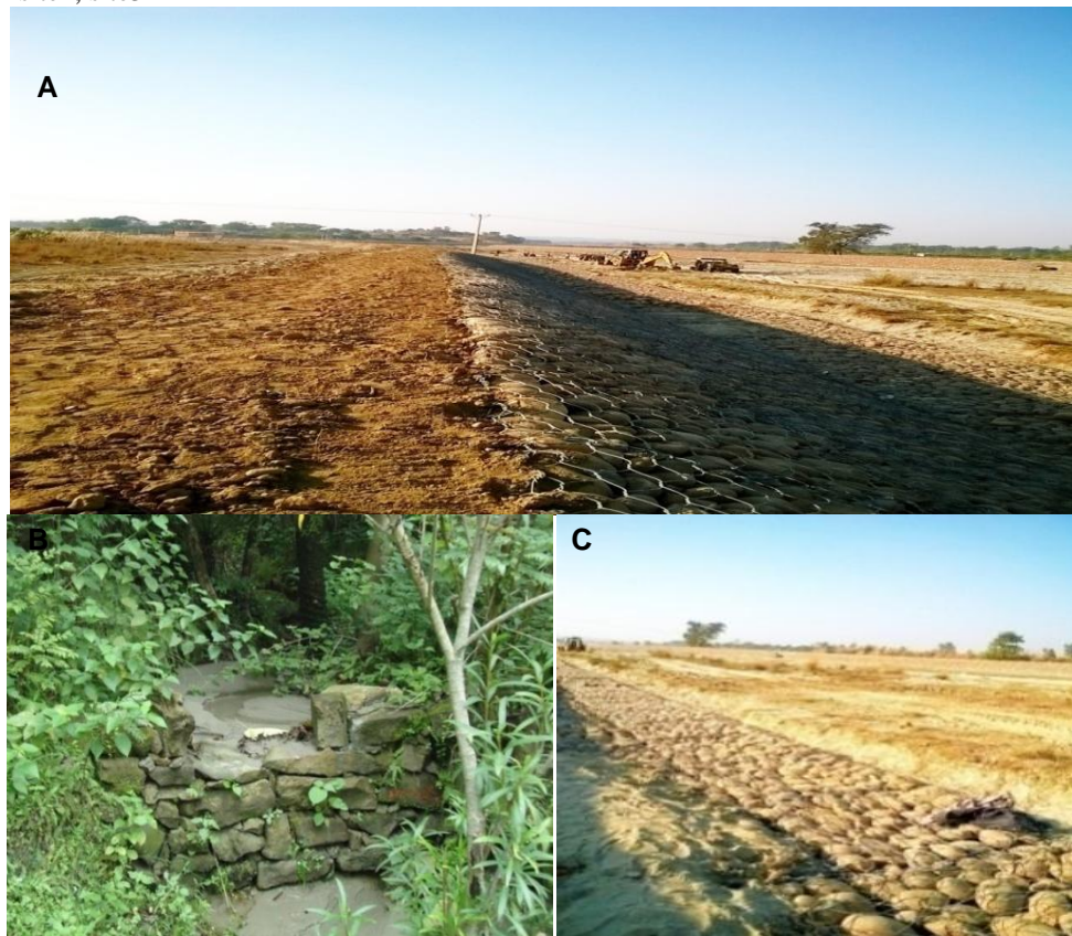
Fig.2; A,swan channelization to control floods and over flow the banks;B-C,crate wire check dams and check dams to save water and soil.
