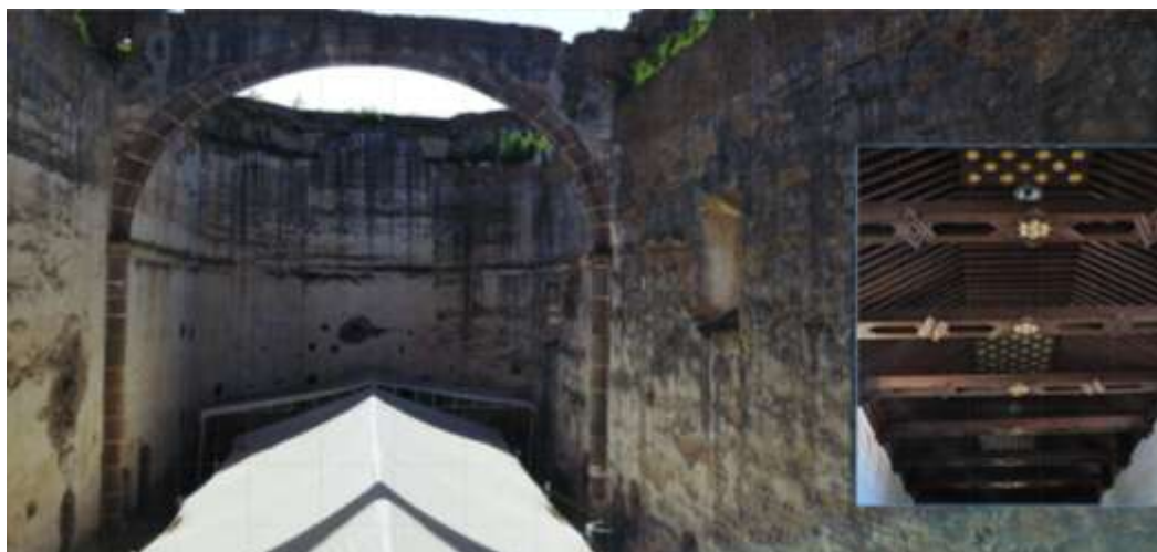
Figure 8. Possible roofing (personal file).
