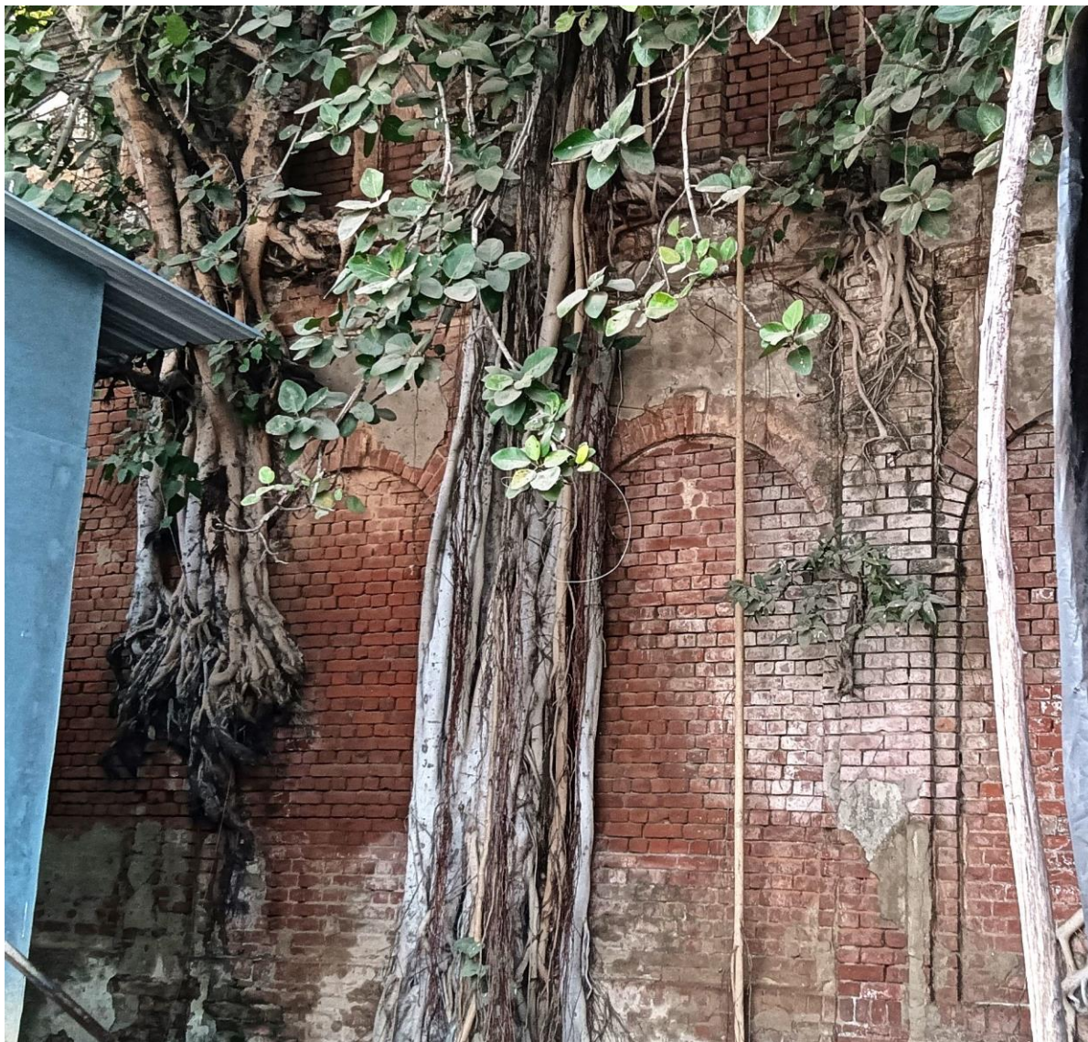
Fig. 2: Banyan tree grown in wall of old building at Lal Kurti, Meerut
