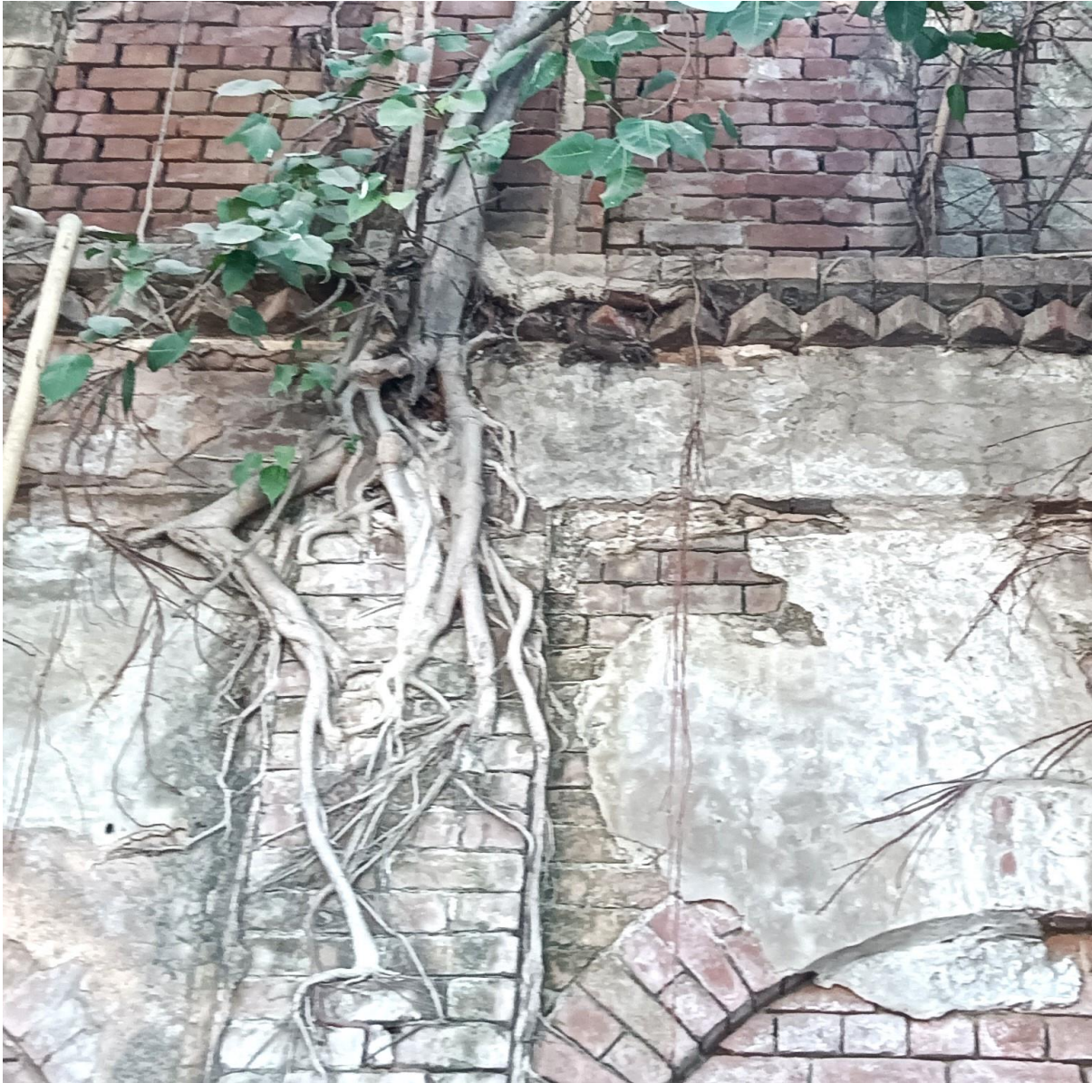
Fig.6: Peepal tree grown in wall of old building at Lal Kurti, Meerut
