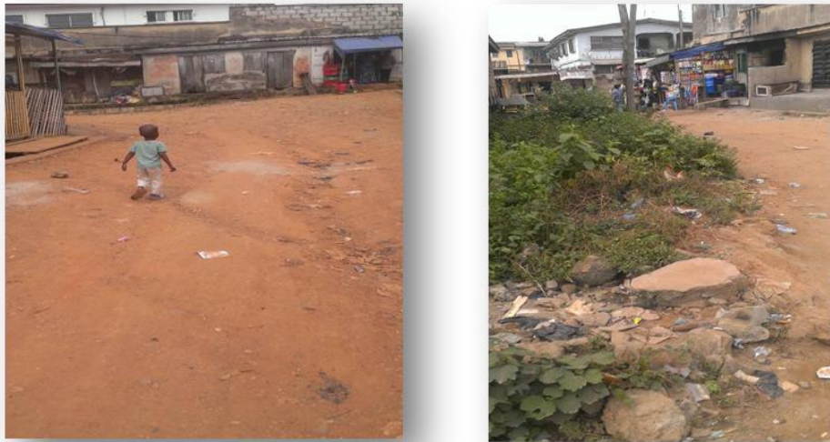
Figure 11: showing roads with no drainage system within study area.
