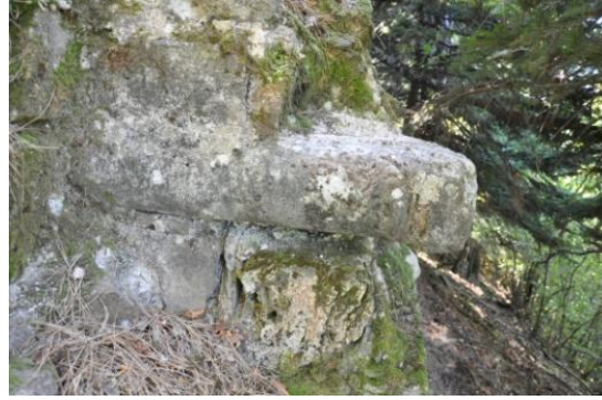
Figure 5 Asarkale, east corner of the tower 1
