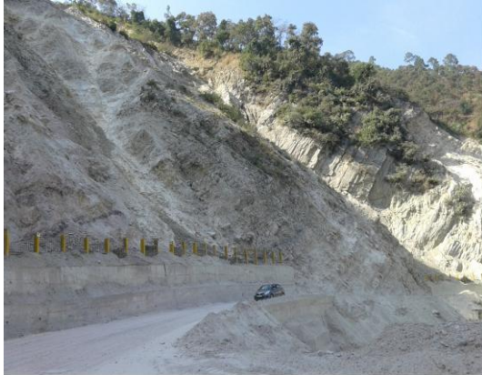
Show retaining wall made by BRO
