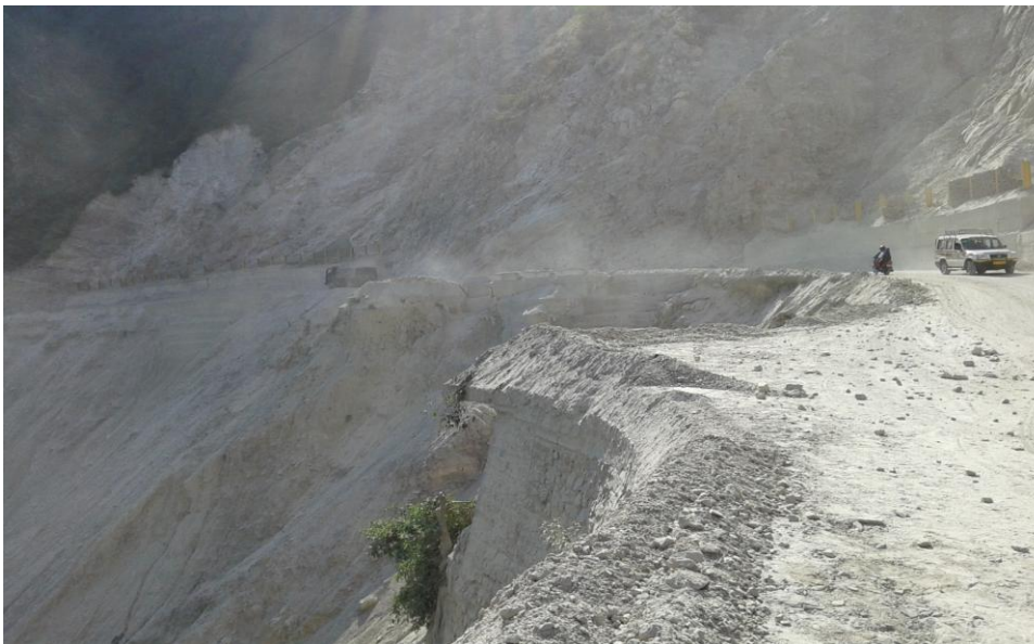
Condition of NH-58 in January 2016
