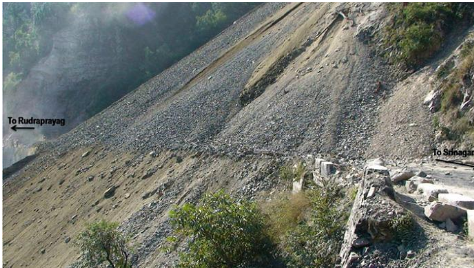
Blockage of the NH-58 due to slope failure in 2013 (Source: Indervir S. Negi, Kishor Kumar, Anil Kathait & P. S. Prasad, 2013)
