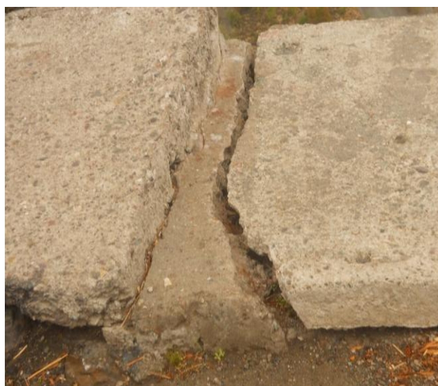
Fig. C. Shows bad condition of retaining walls.
