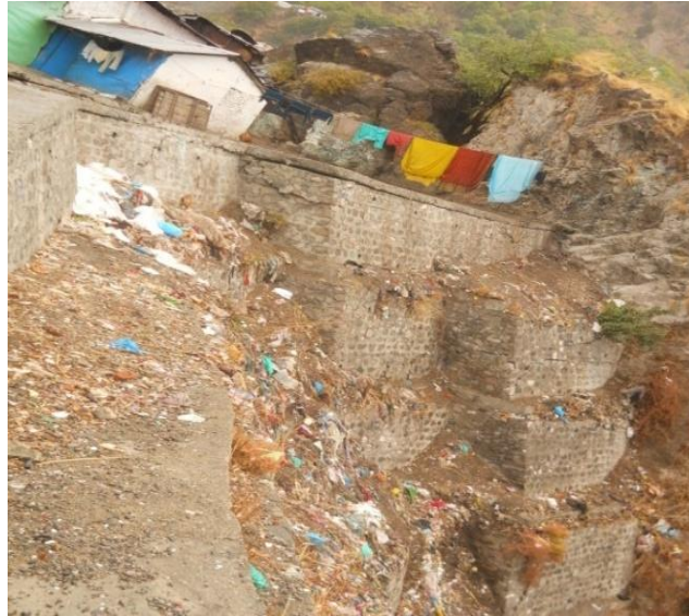
Fig. D. Garbage dumping is the main reason for bad condition of retaining wall
