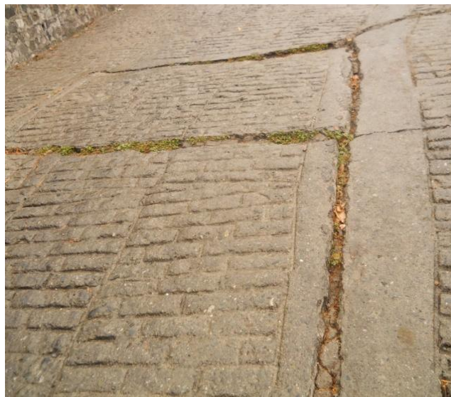
Fig. B. Presents soil creeping through crack in roads.
